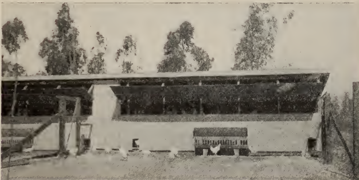
Fig. 8.—San Gabriel type curtain with top tipped out to admit sunlight into house. Plan for the construction of this curtain shown in figure 9.
